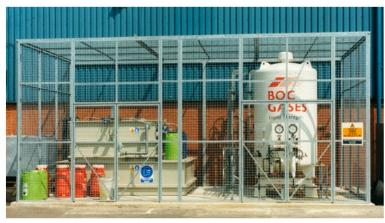
Eurocage is bolted to the floor (from the inside, maintaining security) which means it has the added benefit of being de-mountable and relocated with a minimum of effort. Standard cages are designed around our 1220mm wide panel, however standards configurations do not always fit into the required dimensions. Therefore the non-standard or bespoke design is always an option.
